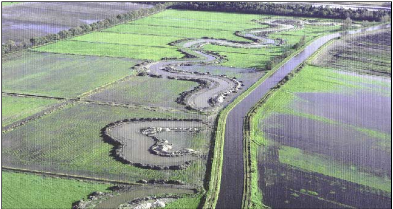
Artificial Meanders - Work going on in Germany to restore meanders to the Rhine. The object is to reduce flooding in the Netherlands (source: IRMA Secretariat, The Netherlands).
