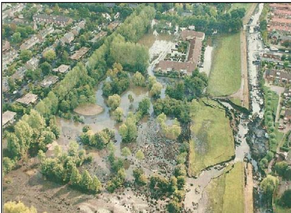
Flooding in Amsterdam- this took place in July 2003 and was due to drought which caused cracks in the earth and peat embankment resulting in failure.
