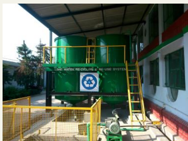
Lime water recycling and reuse system Kanpur leather tannery ©WWF-UK/Conor Linstead
