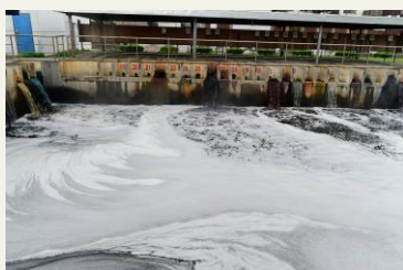
Wastewater collection tank in the Industrial Park's wastewater treatment plant, China ©A Tu
